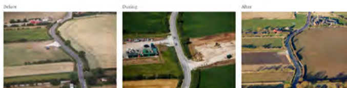
Example of cable route construction from a previous project (Titchin Knoll)
